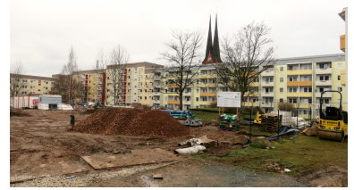
Baustart am Alberti-Park
